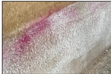
Finished Seal Coat
