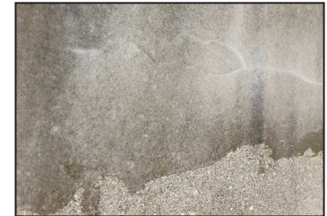
Finished Glaze Coat
